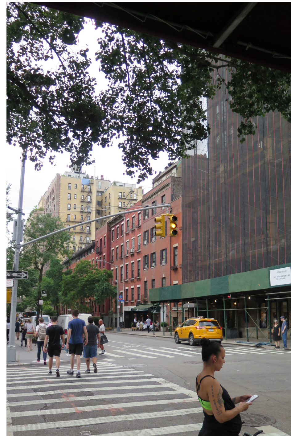
6. STREET VIEW LOOKING NORTH FROM UNIVERSITY PLACE INCLUDING MOCK UP CONSTRUCTION (MOCK UP NOT VISIBLE)
