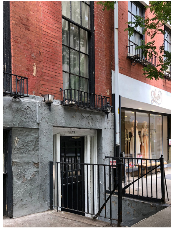
1. EXISTING ENTRY WAY AT E 9TH ST
