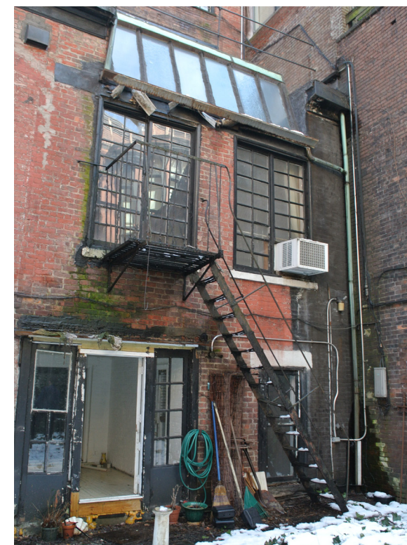
4. EXISTING REAR FACADE NW CORNER, BASEMENT & 1ST FLOOR
