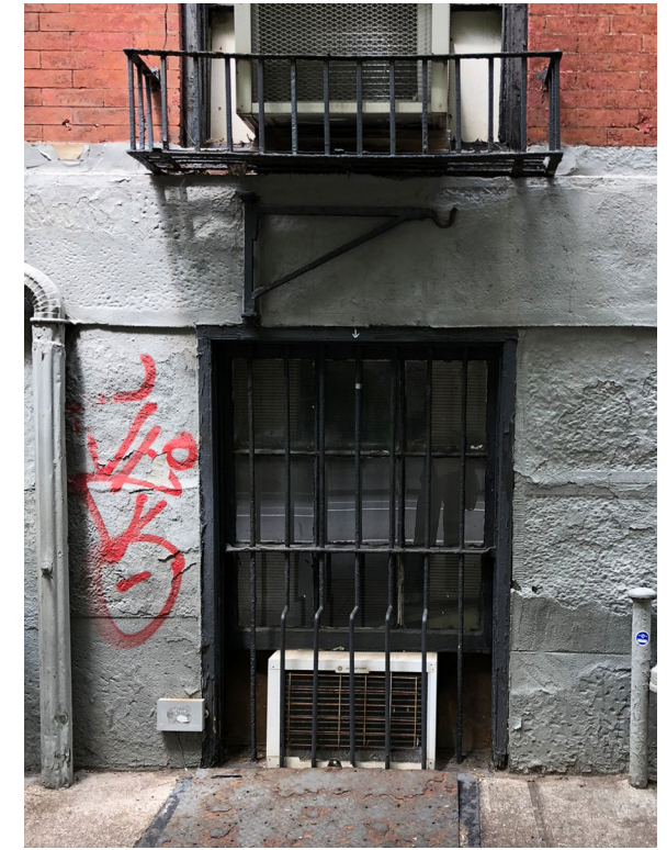
4. EXISTING WINDOWS AT BASEMENT
