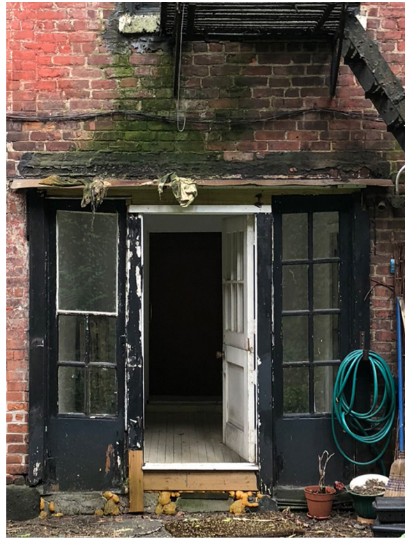
2. BASEMENT, DOOR TO REAR YARD
