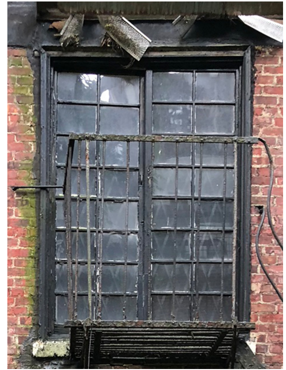
4. 1ST FLOOR, DOOR TO FIRE STAIR
