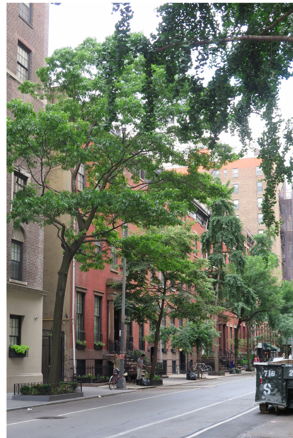
10. STREET VIEW LOOKING EAST FROM E 9TH STREET INCLUDING MOCK UP CONSTRUCTION (MOCK UP NOT VISIBLE DUE TO OBSTRUCTING TREE)
