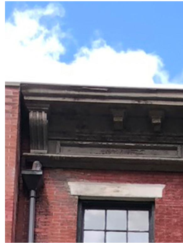
7. EXISTING CORNICE S/W CORNER
