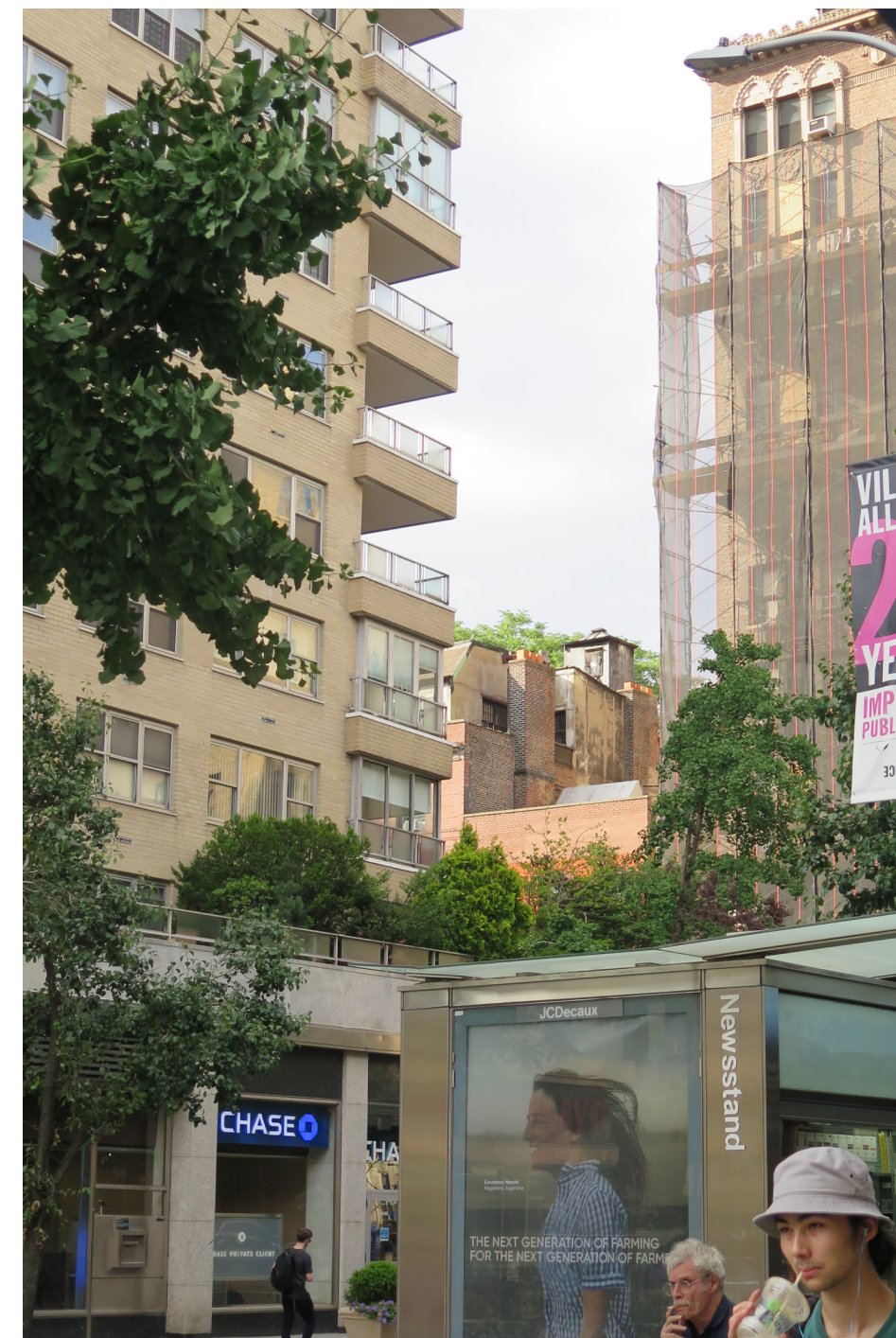
2. STREET VIEW LOOKING NORTH FROM UNIVERSITY PLACE INCLUDING MOCK UP CONSTRUCTION (BUILDING NOT VISIBLE)
