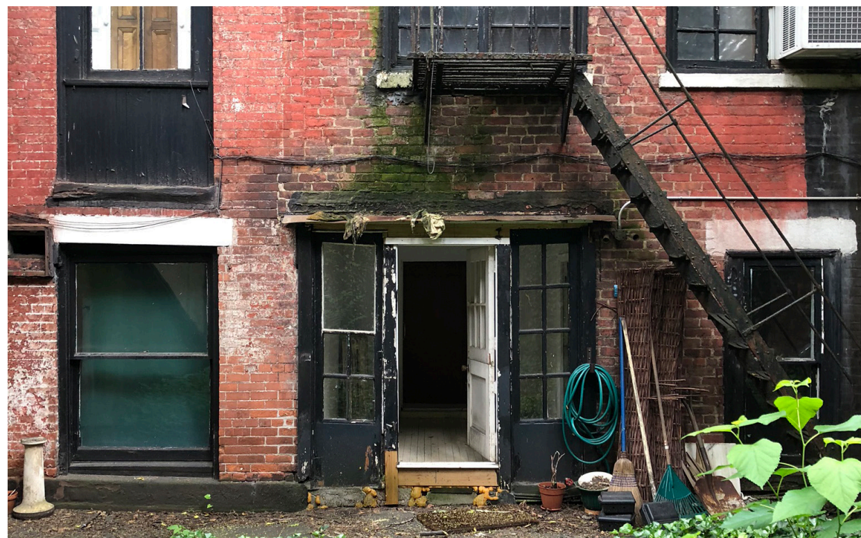
3. EXISTING REAR FACADE, BASEMENT & 1ST FLOOR
