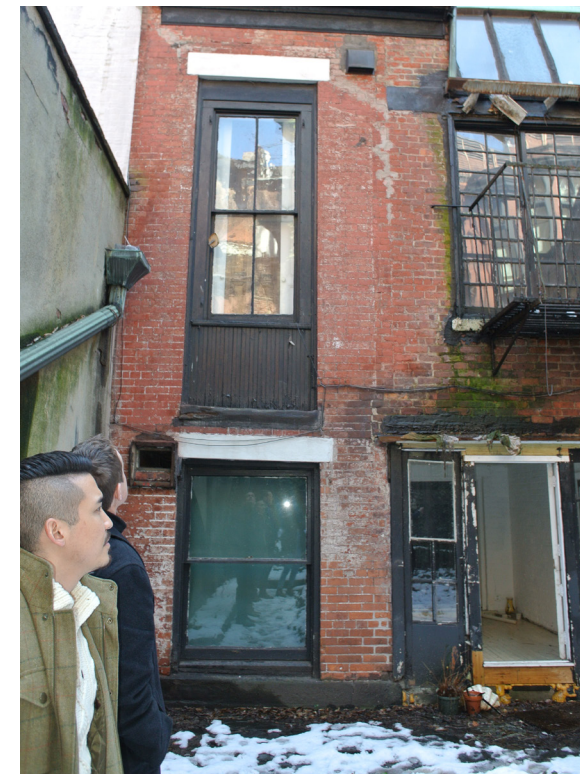
2. EXISTING REAR FACADE NE CORNER, BASEMENT & 1ST FLOOR
