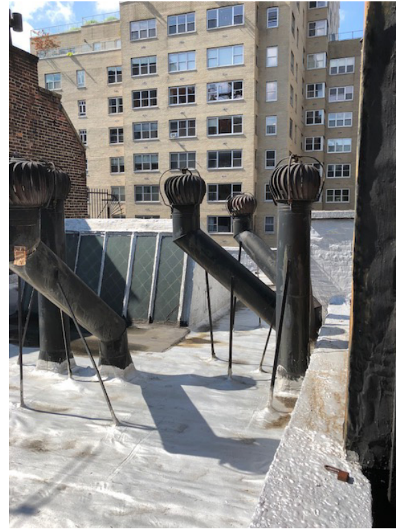
2. EXISTING EXHAUST FLUES
