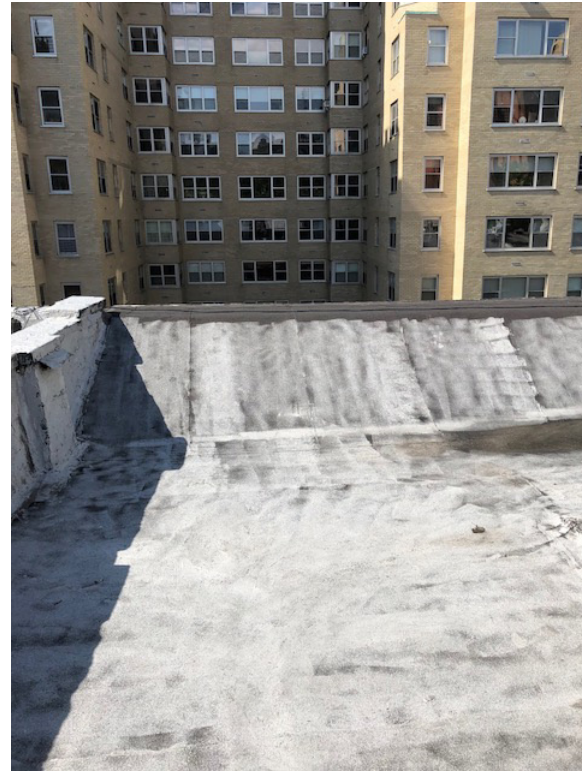
1. EXISTING ROOF PARAPET
