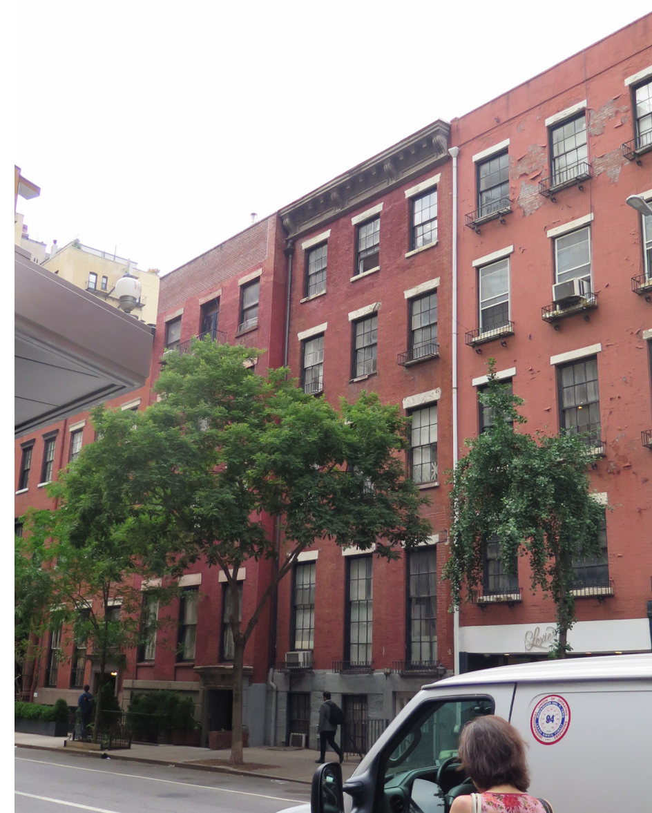
18. STREET VIEW LOOKING NORTH FROM E 9TH STREET INCLUDING MOCK UP CONSTRUCTION (MOCK UP NOT VISIBLE)
