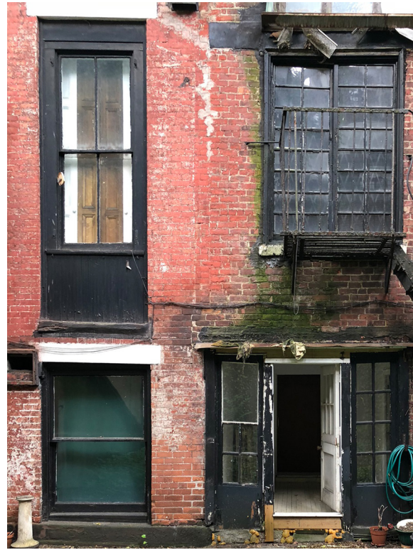
1. BASEMENT & 1ST FLOOR NE CORNER WINDOWS
