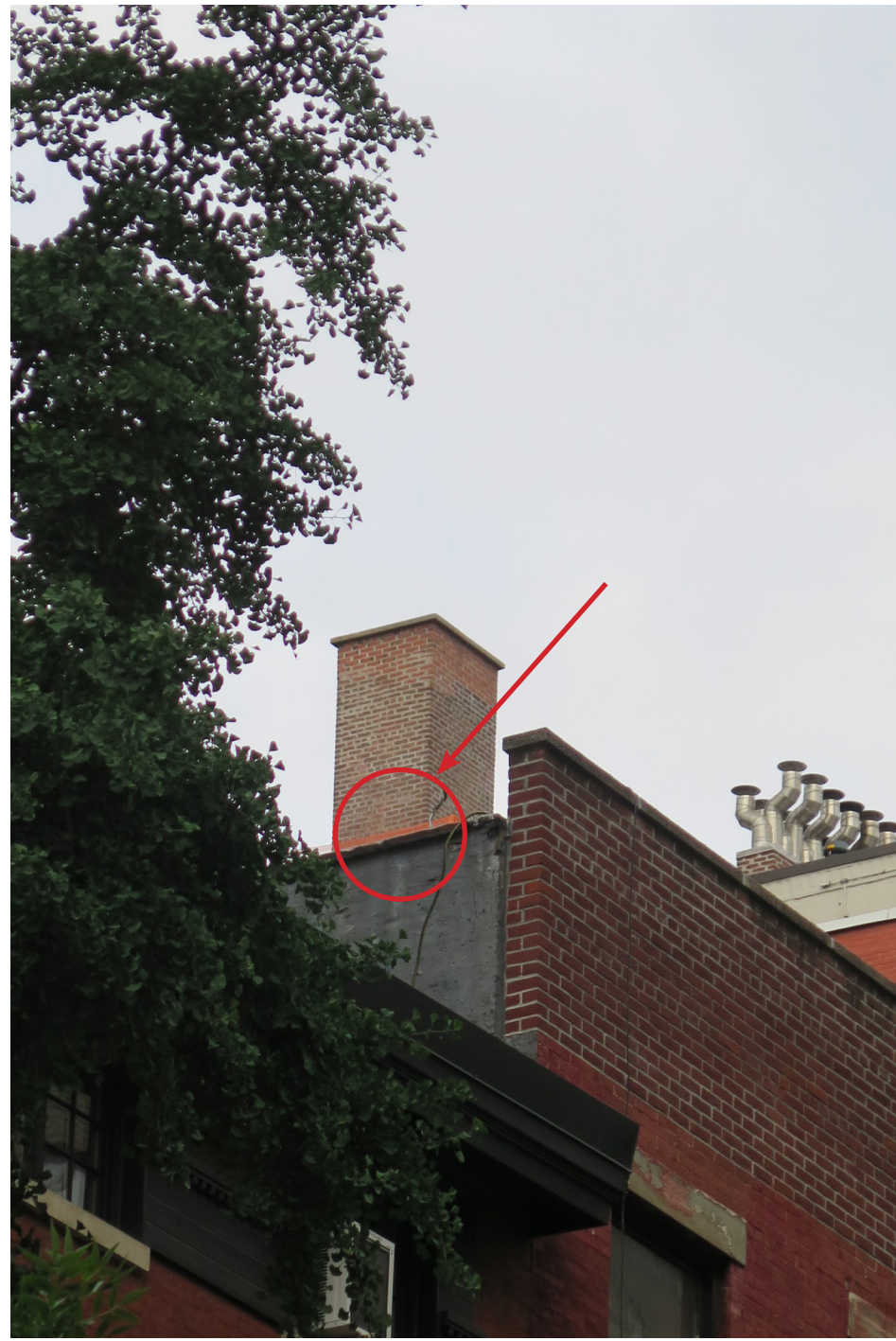
14. ENLARGED STREET VIEW LOOKING EAST FROM E 9TH STREET INCLUDING MOCK UP CONSTRUCTION
