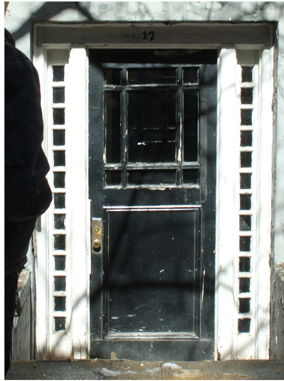
2. EXISTING ENTRY DOOR AT E 9TH ST
