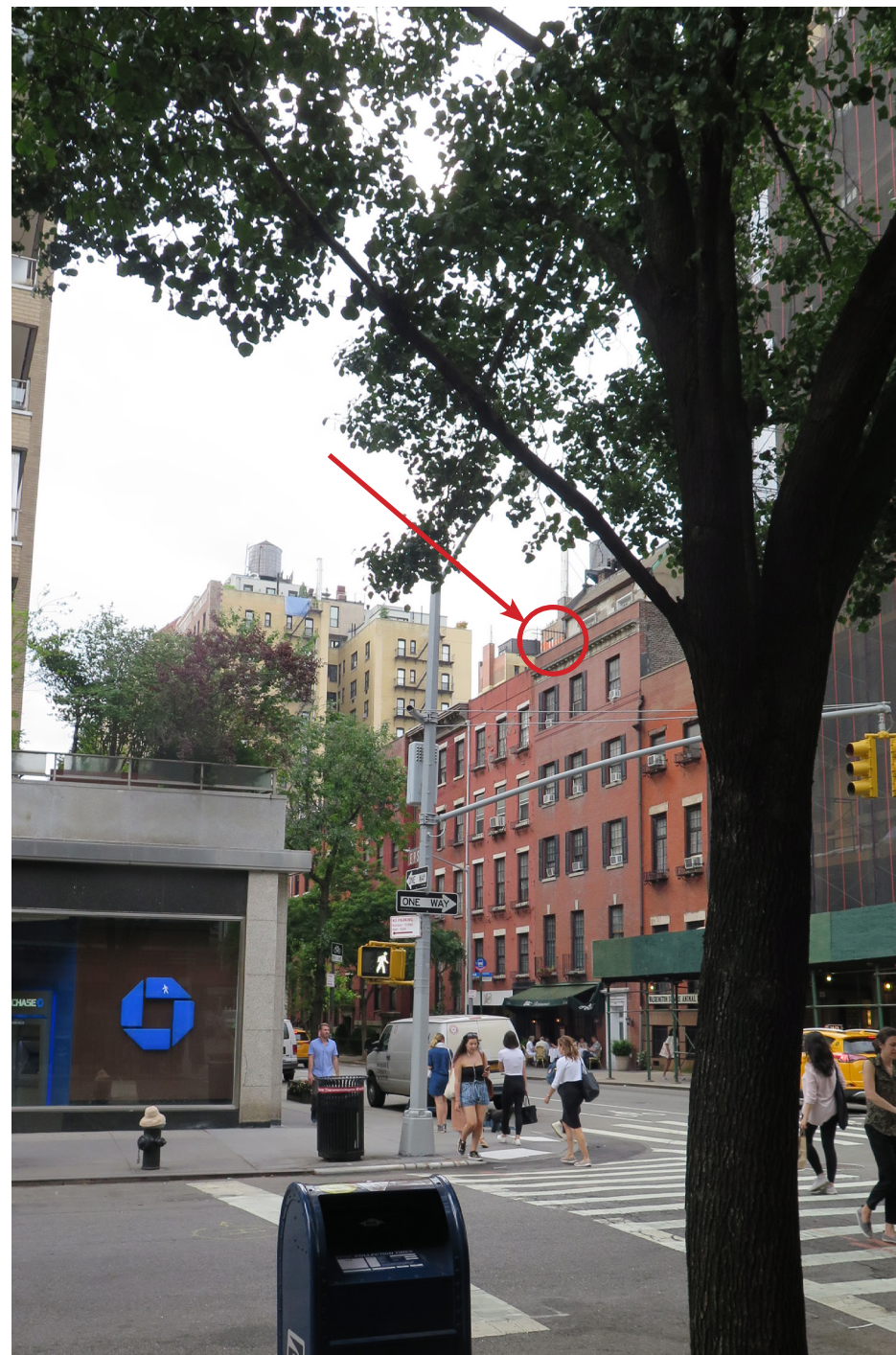
5. STREET VIEW LOOKING NORTH FROM UNIVERSITY PLACE INCLUDING MOCK UP CONSTRUCTION (MOCK UP NOT VISIBLE)
