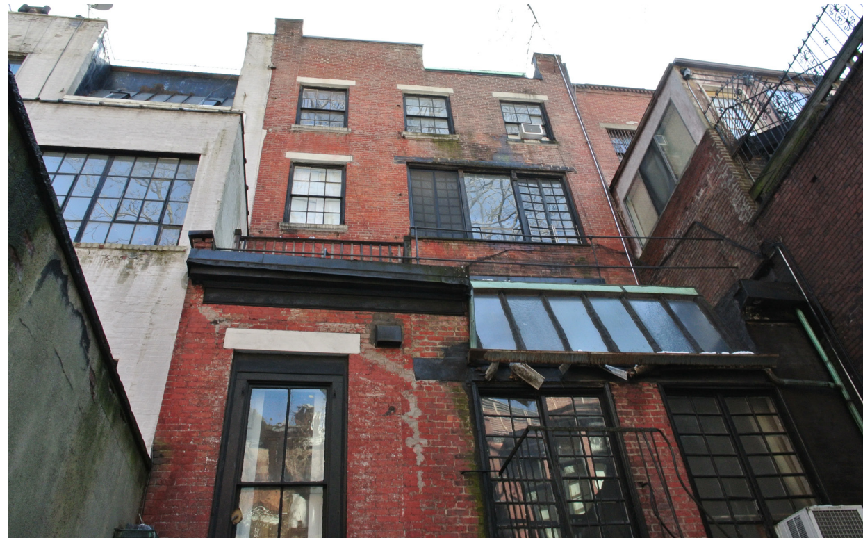
1. EXISTING REAR FACADE, FLOORS 1-4
