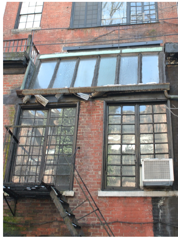
5. 1ST FLOOR, SKYLIGHT
