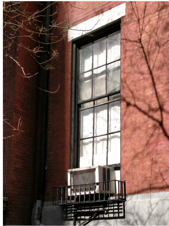
5. EXISTING WINDOWS AT FIRST FLOOR
