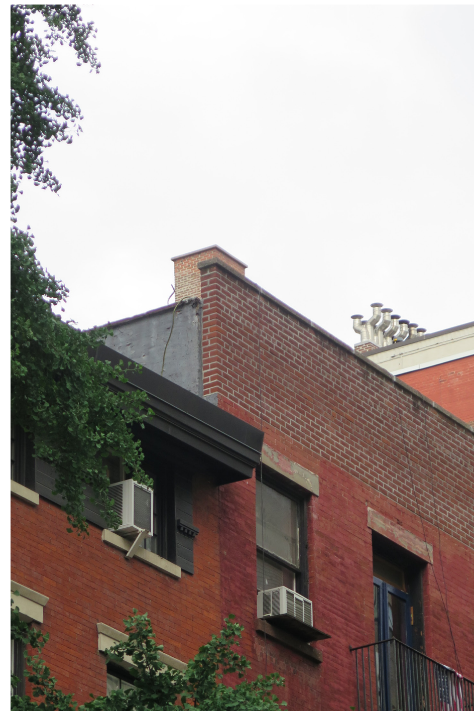
16. ENLARGED STREET VIEW LOOKING EAST FROM E 9TH STREET INCLUDING MOCK UP CONSTRUCTION (MOCK UP NOT VISIBLE)
