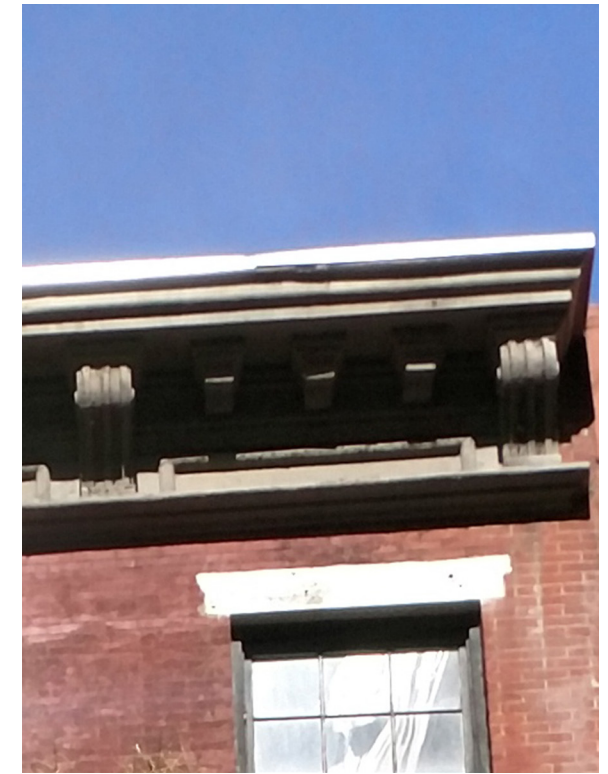
8. EXISTING CORNICE S/E CORNER
